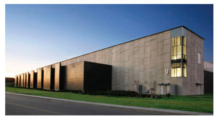
PARADIGM was selected as the engineer of record for this 126,569 gsf two-story LEED certified building. This structure, housing office and customer support areas, computer rooms and electrical and mechanical equipment rooms, is supported on auger cast displacement piles at depths of up to  $50^{\circ}-60^{\circ}$ , with the tops of the piers and caps interconnected with bi-directional grade beams. The first-floor slab is supported on grade, above the grade beams and pier caps.
